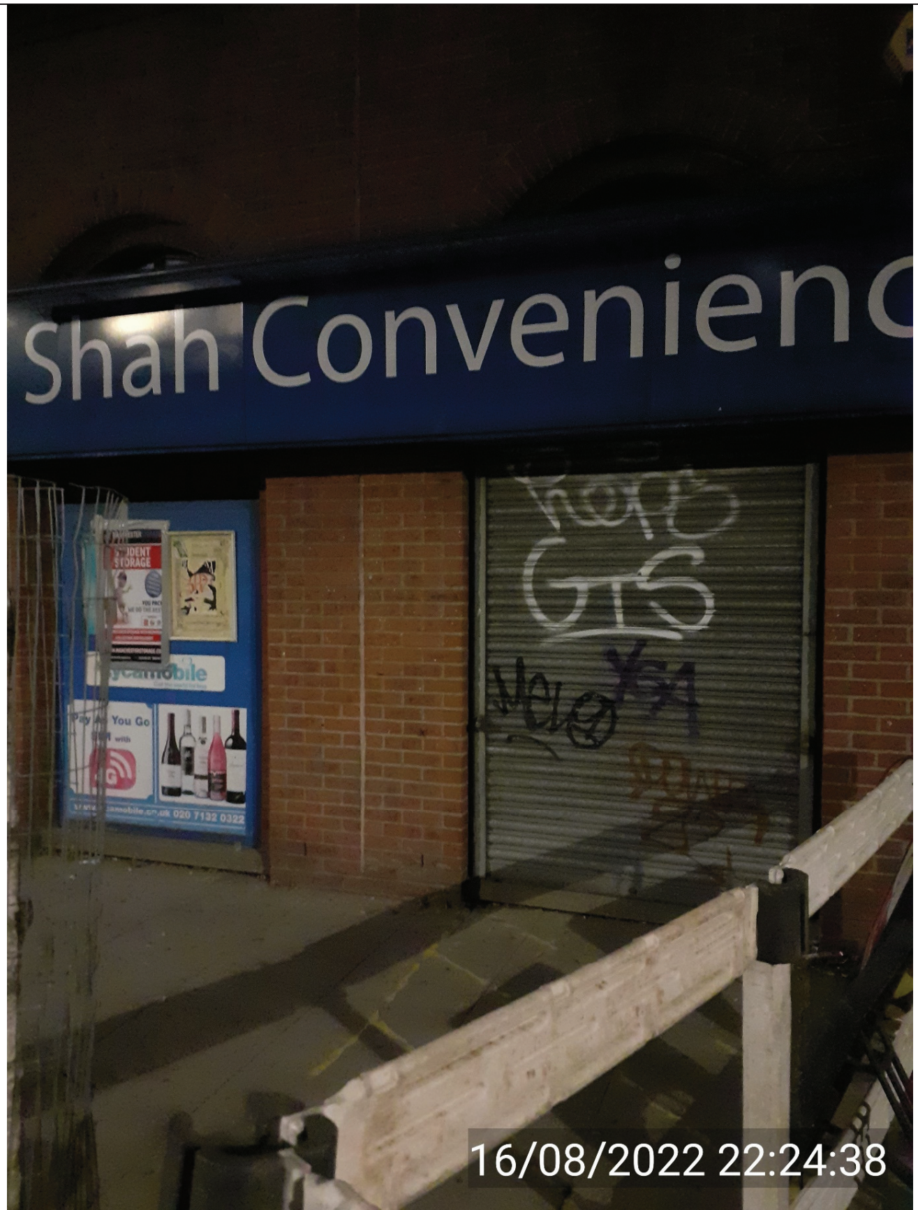
Shah Convenience Store – Chester Street elevation.
